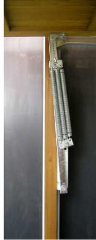
High lift spring system to maximise drive through space for most family cars
